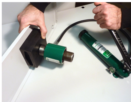
Making the cut-out with a punch.
