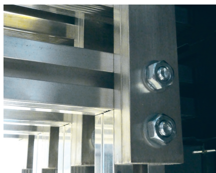
Connection between an aluminium busbar and a double main busbar created using aluminium bars.
