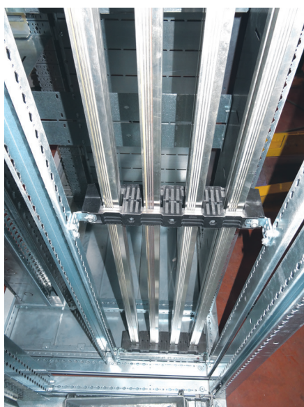
Position the busbars and tighten the supports to ensure the bars are held in place. (Tightening torque: see page 27).
